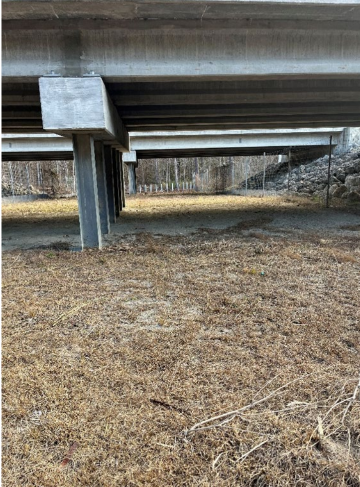
Figure 16. Wildlife underpass on US 17 in Jones County for connecting habitat for a range of species.
